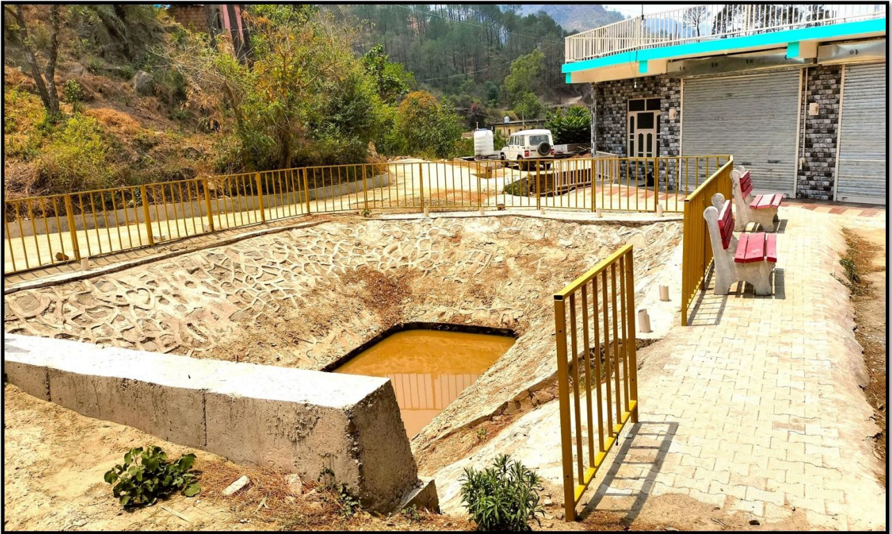
Figure 9 Enhancement of Pond at Km. 43+760 (RHS)
