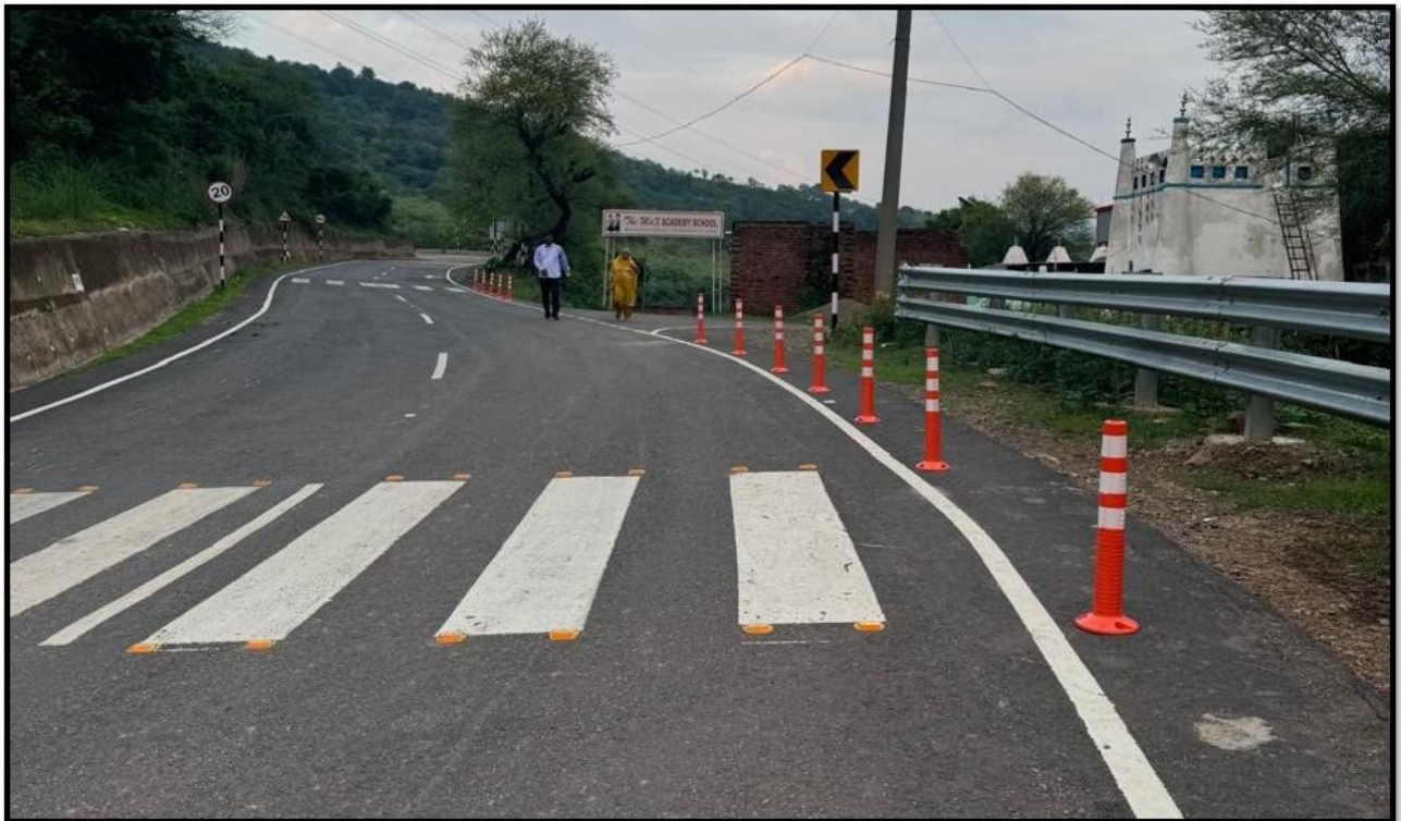
Figure 1 Installation of Spring post at Km. 12+940 near School
