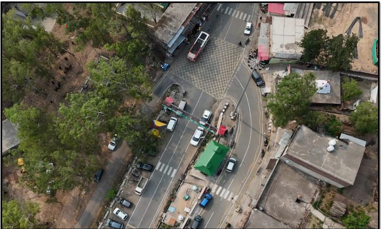
Figure 10 Ramshahar Junction Km. 44+733
