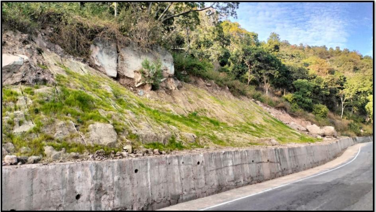
Figure 5 Slope stabilization work with bioengineering practices Jute netting at Km. 18+440 (LHS)
