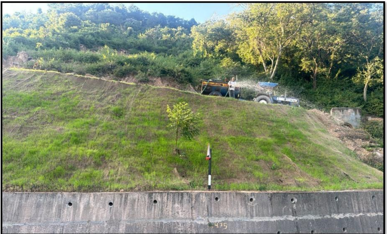
Figure 8 Slope stabilization by Jute netting work at Km. 17+250 (RHS)
