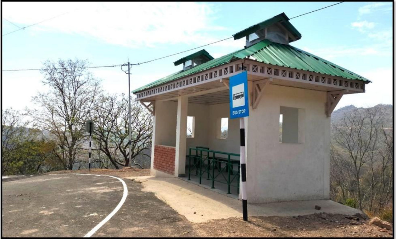
Figure 7 Bus shelter at Km. 35+040 (LHS)
